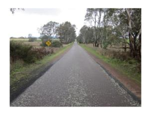
Whilst a narrow seal with well-maintained shoulders is acceptable for tourist traffic, each municipality may wish to implement a program to upgrade the seal width to 6.0m over a number of years.
