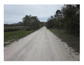
It is considered a 4.0m seal with 1.5m shoulders is a satisfactory pavement, particularly given the route includes 35 km of existing narrow seal roads.
